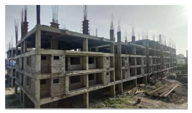
Block A2: Fourth Floor level slab concrete casting 100% completed.
